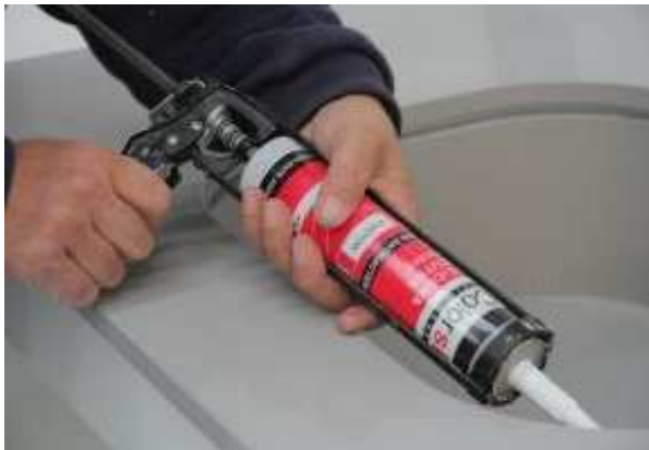
6. Securing the kitchen sink to the worktop with silicone resin.
